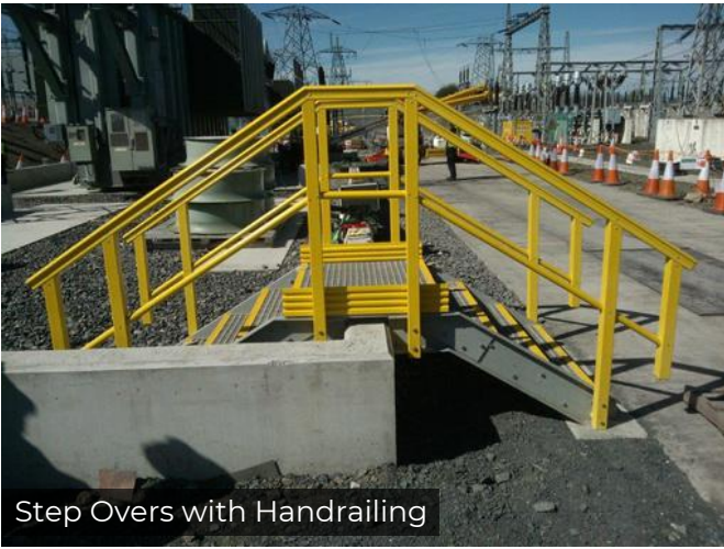
Rooftop Access Walkway and Step Overs
