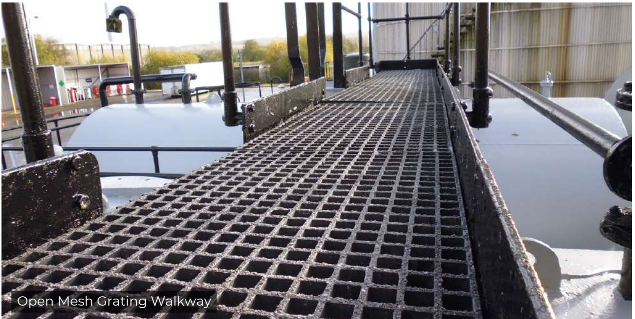
Raised Rooftop Walkway for Disability Access
